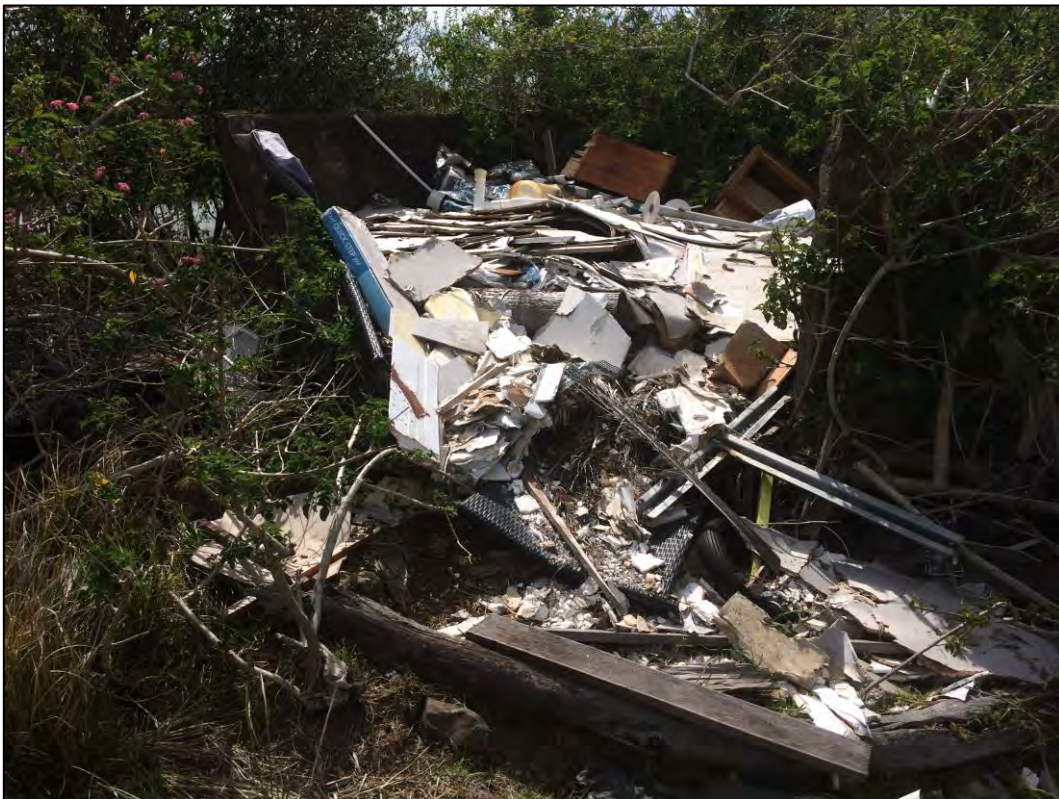
Photograph 12 – Stockpile of demolition waste containing bonded asbestos fragments, identified in the eastern portion of the site, as observed on the 12.11.201
