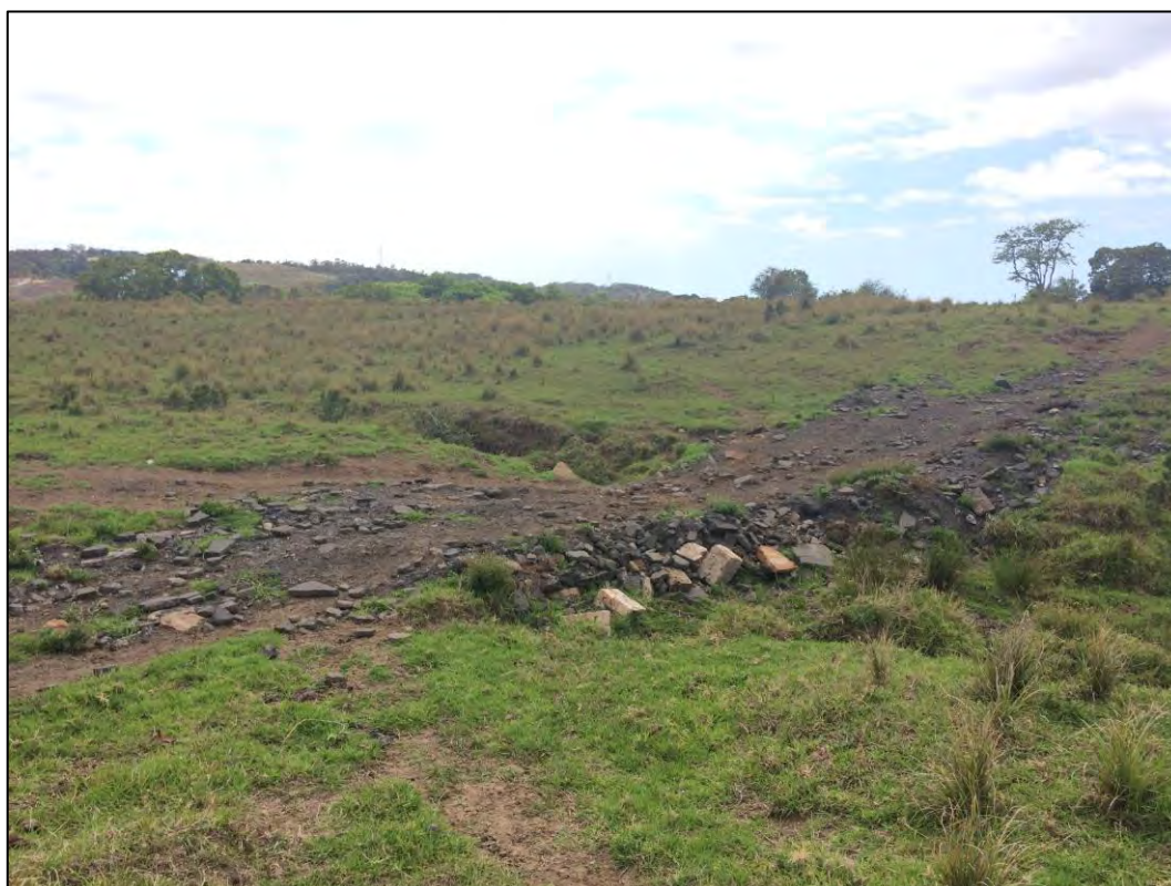
Photograph 4 – Imported fill material used as a crossing, as observed on the 12.11.2018
