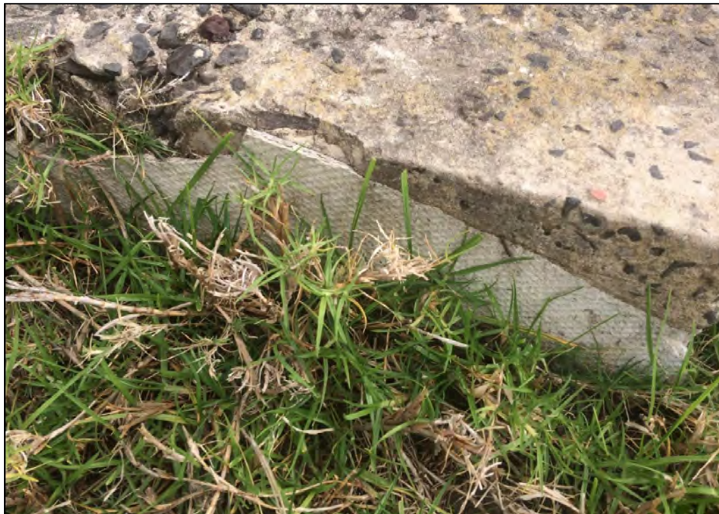
Photograph 14 – Suspected ACM sheeting attached to one of the concrete footings in the eastern portion of the site, as observed on the 12.11.2018
